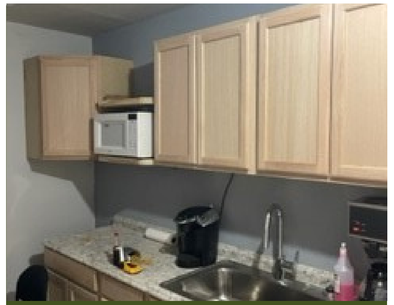
PARKS BUILDING CABINET INSTALL AND PAINTING
